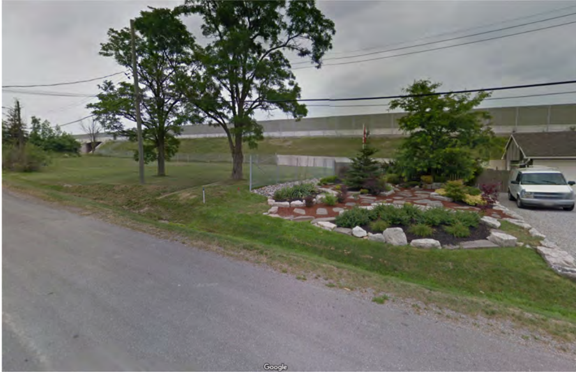
View of Highway 6 from Atkinson Road.
