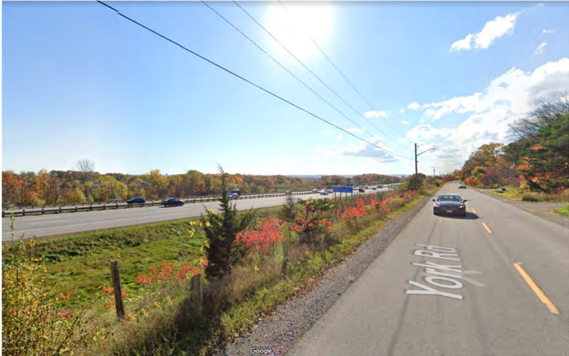
View of Highway 403 from York Road, looking south
