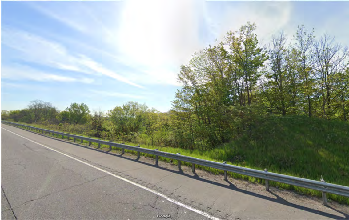
View of slope to RBG from Highway 403
