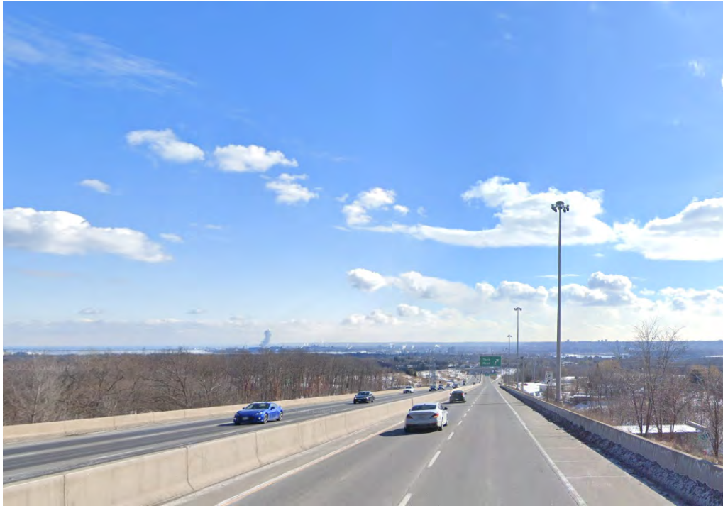
View south along Highway 6 towards Lake Ontario.
